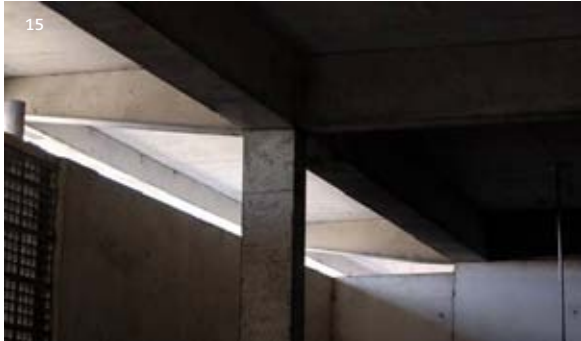
FIGURE 15 Pillar head double tee junction.
