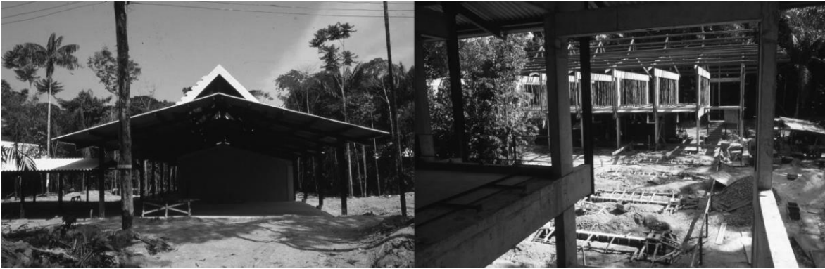
IMAGE 5 - UFAM: building process.
